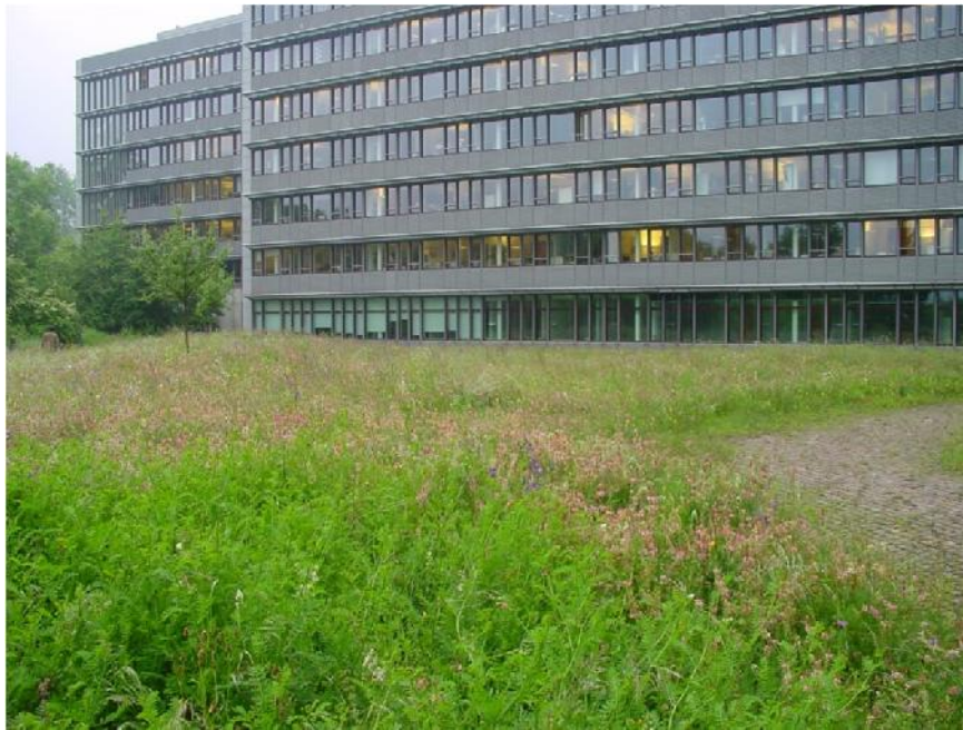
Zentrale, Credit Suisse in Zürich
